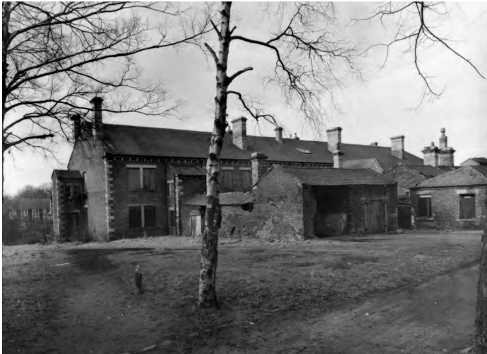
FIG. 1. Brampton Workhouse in 1958 prior to demolition Carlisle Image Bank: ct04535 .
